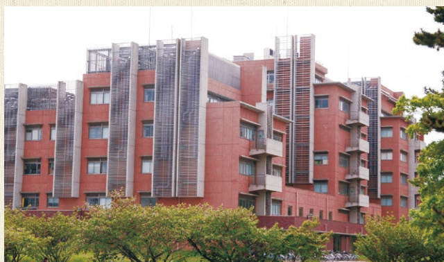
物質生産棟 (左) と生命環境棟 (右) [Material Science and Technology Building (left), and Life Science and Environmental Science Building (right)]
